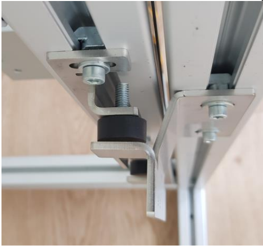
Figure 6: Doorstop on back side of swinging door
